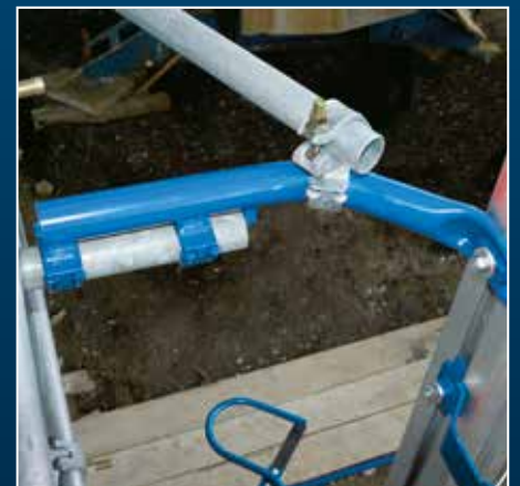
Anchoring on scaffolding
