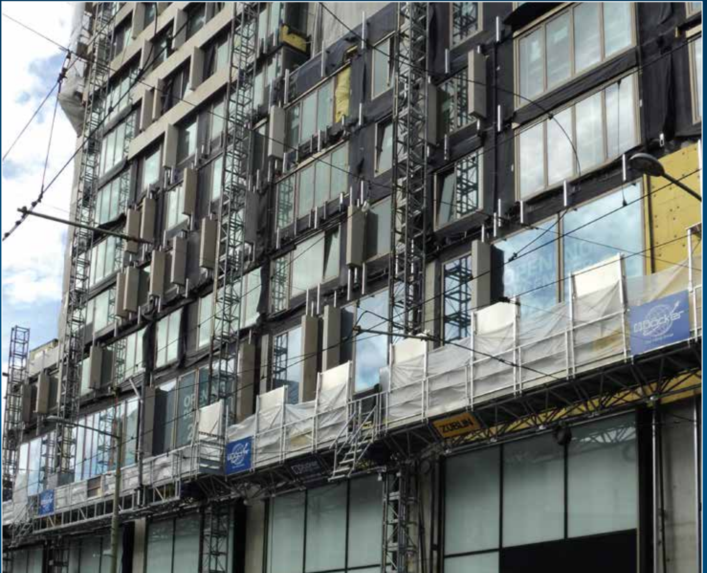
Modular design of the Böcker Maxi-Climber
