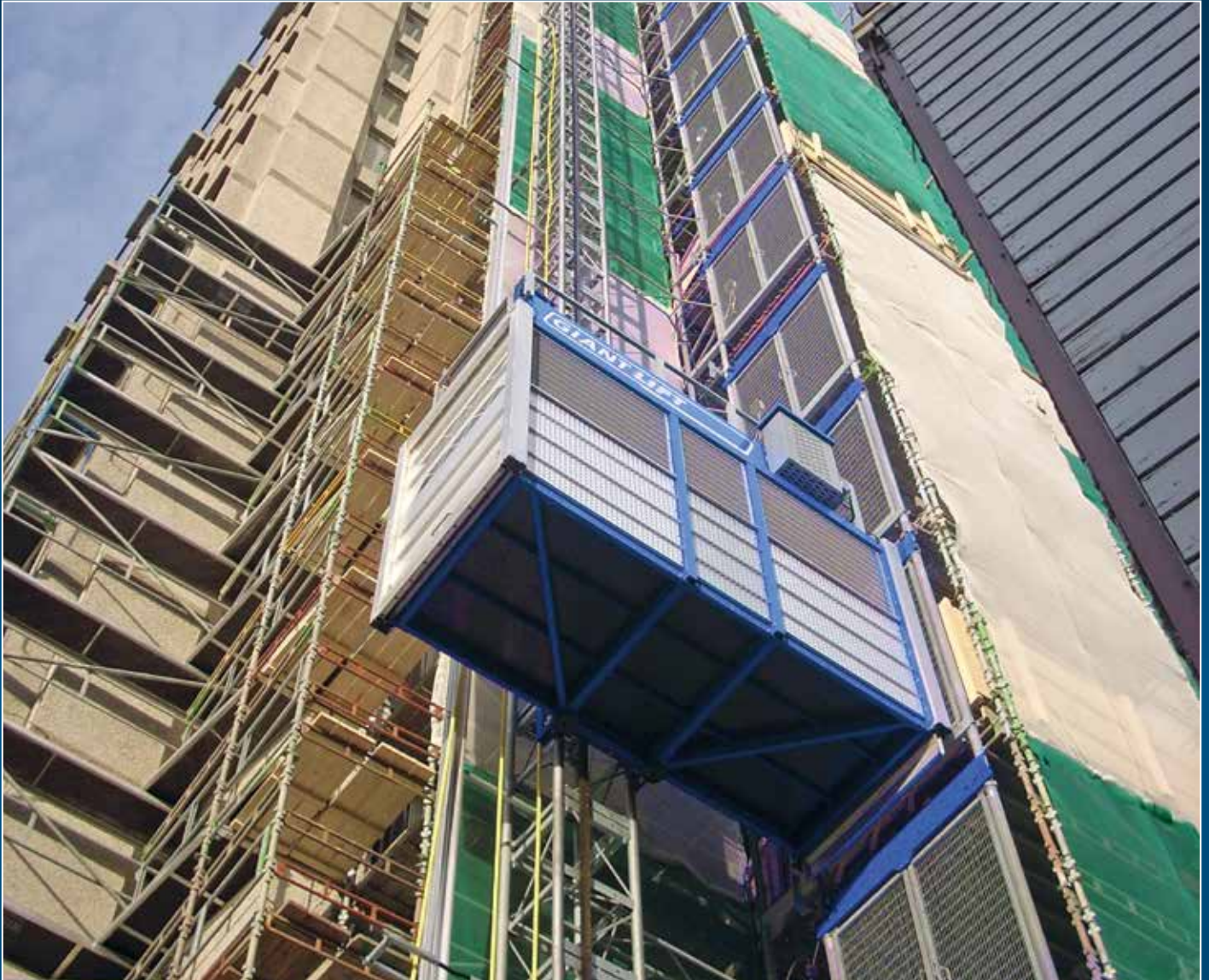
GIANT-Lift – installation with landing scaffolding
