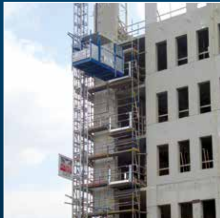
Superlift LX 2024 – A34 in single-cage operation
